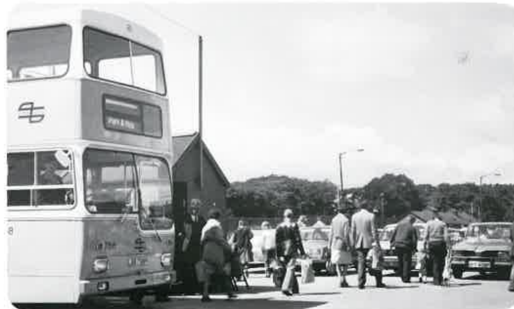
Park-and-Ride by bus is already popular with motorists and now Metro will extend this by giving Park-and-Ride facilities at many stations.
