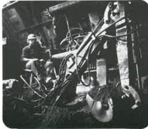
Work on the Metro tunnels is now nearing completion.
