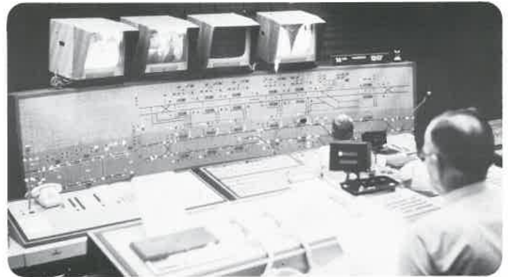
The interior of the Control Centre will be similar to this one in Germany.
