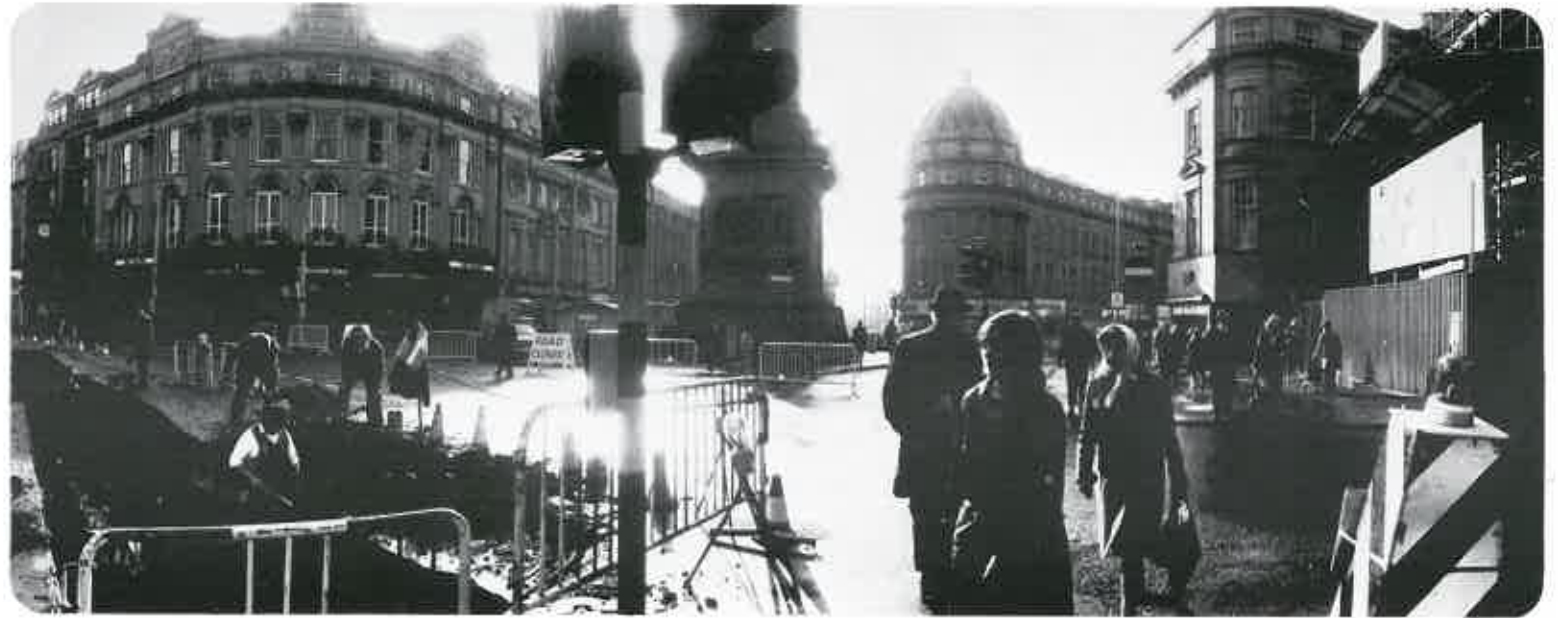
Building Metro is bound to cause some disruption but great effort is made to keep this to a minimum.
