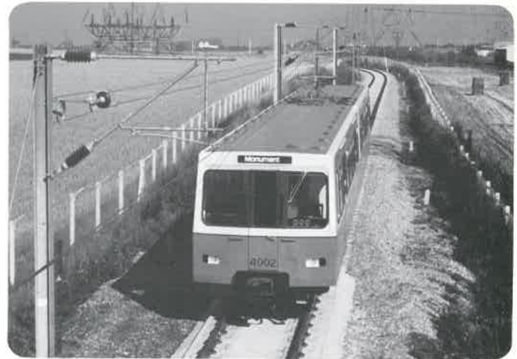
Different types of track bed are being tried out at the Metro Test Track.
