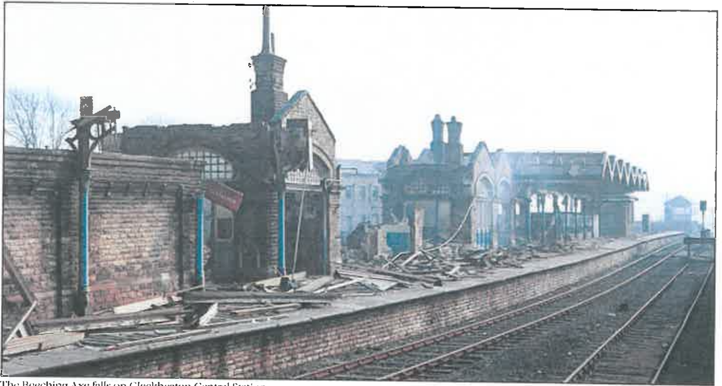
The Beeching Axe falls on Cleckheaton Central Station
