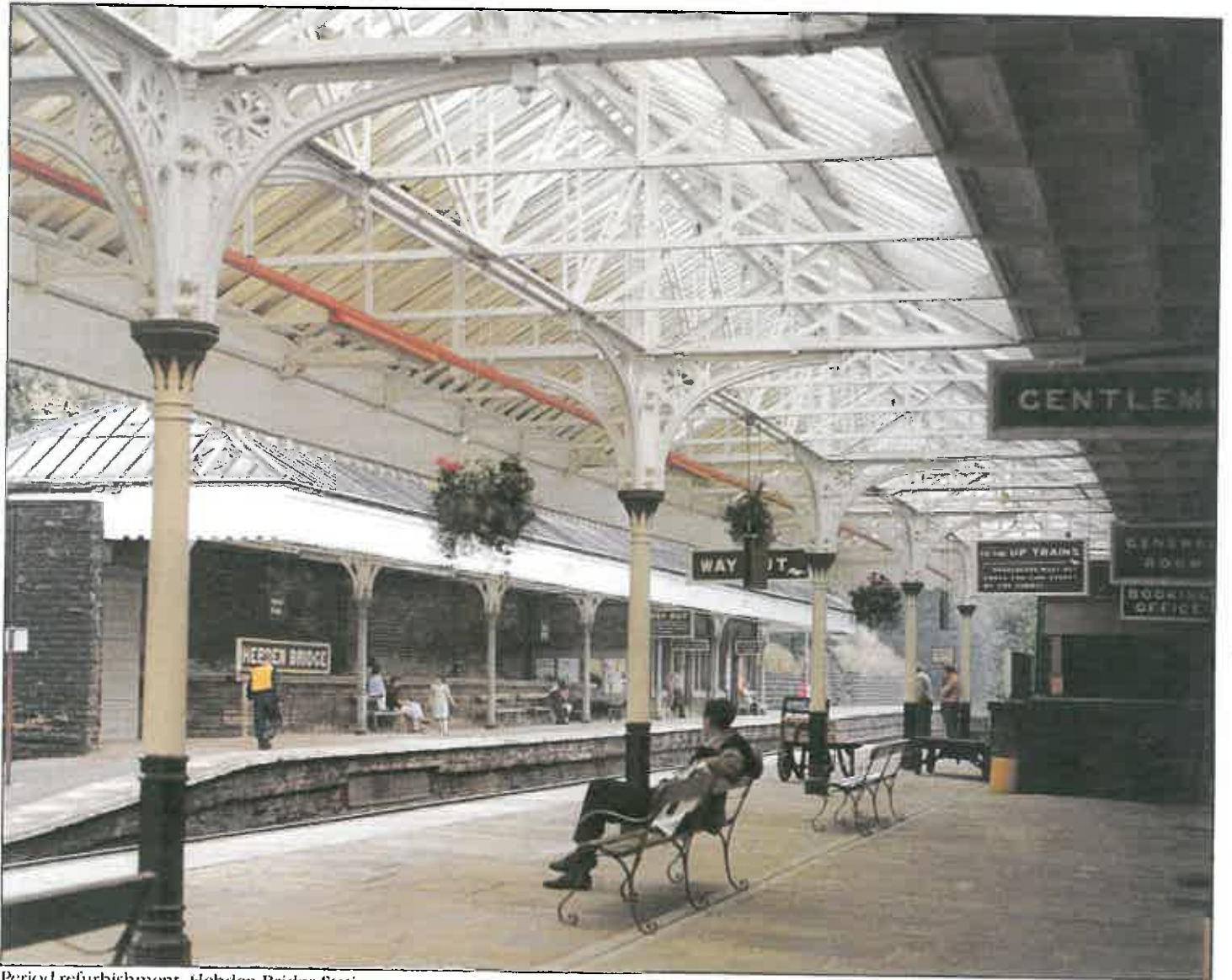
Period refurbishment, Hebden Bridge Station
