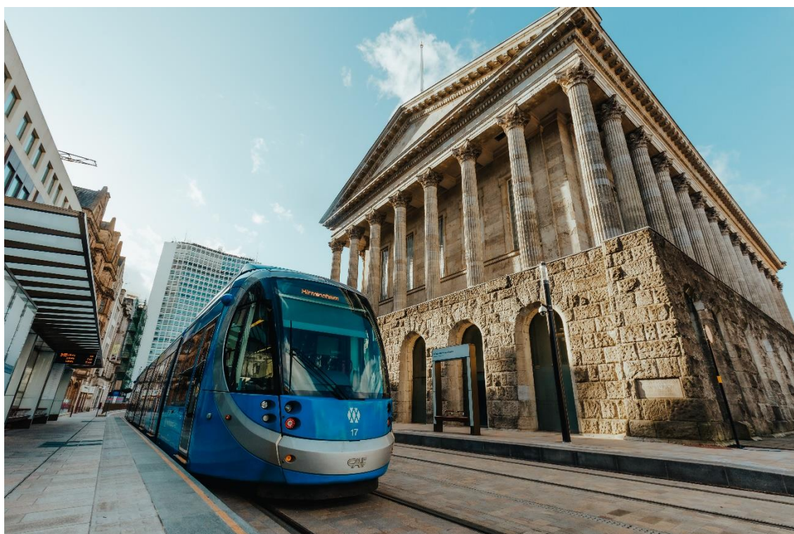
Figure 6.3: West Midlands Metro and Birmingham Town Hall– Catenary Free Operation in Victoria Square, Birmingham
